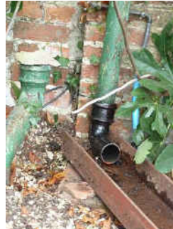
Downpipe Disconnection
